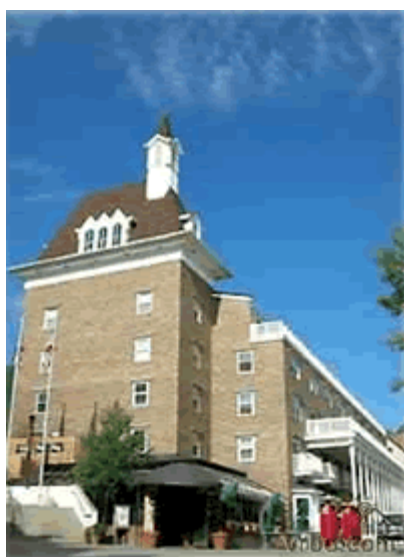
Silver Mill House Building
